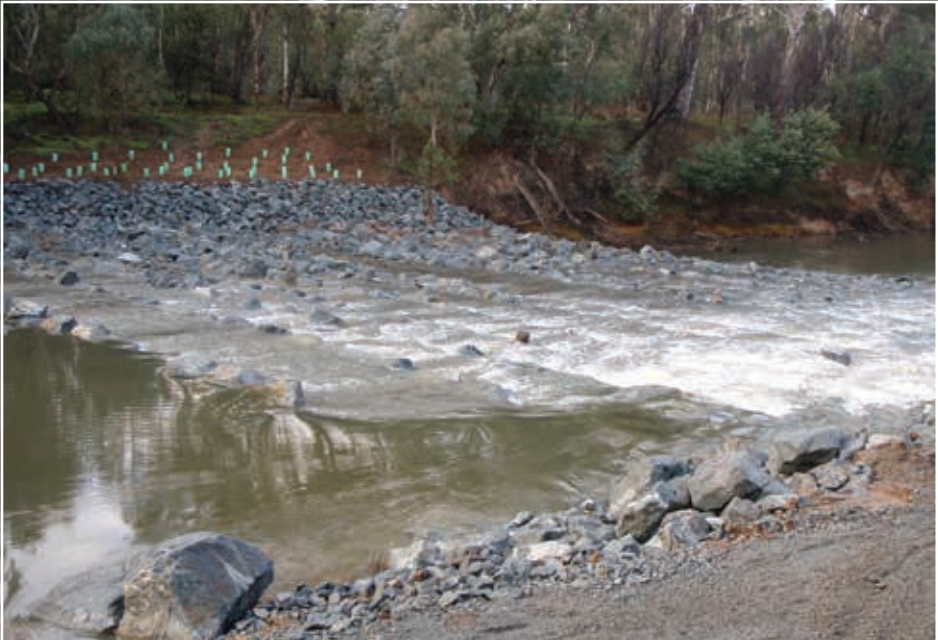
▲ Fishway constructed to replace the Shepparton weir.
