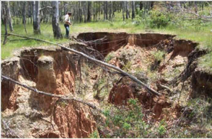
◀ Lowered water quality - erosion and associated sedimentation
