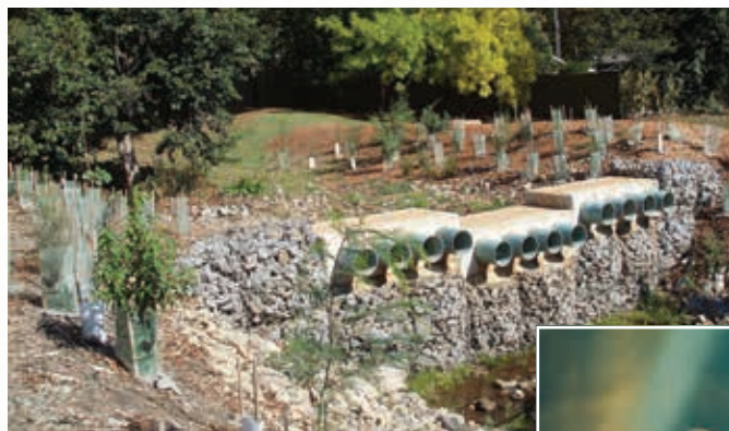
▲ Trout barriers to prevent trout moving upstream into Barred galaxias habitat in Marysville.
