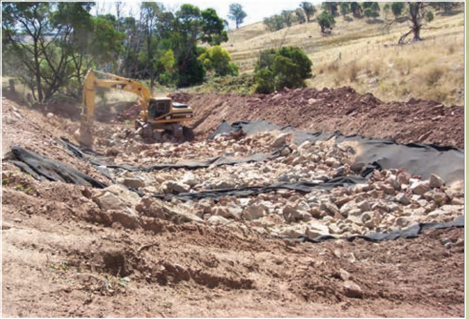
▲ Erosion control works underway.
