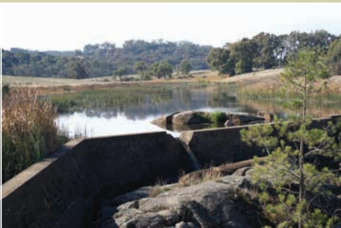
◀ Barriers - man made structures impeding fish migration
